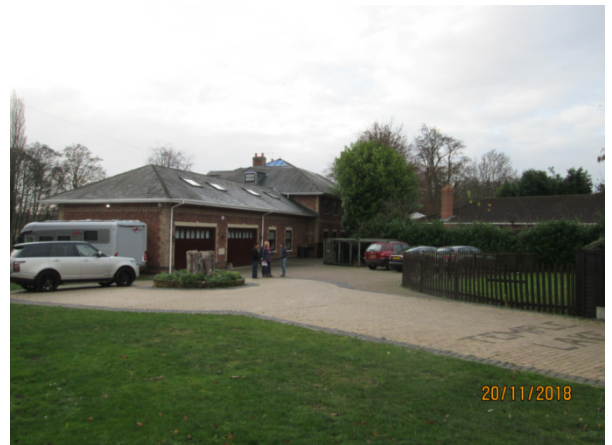
Proposed location of garage and relationship with the host dwelling and the west boundary (adjoining The Old Orchard).
